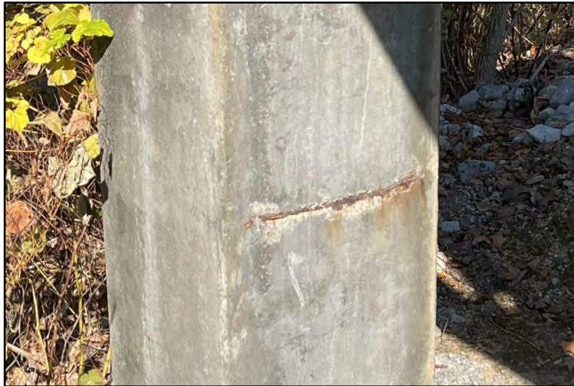
Image 11: Concrete Pier Spall
