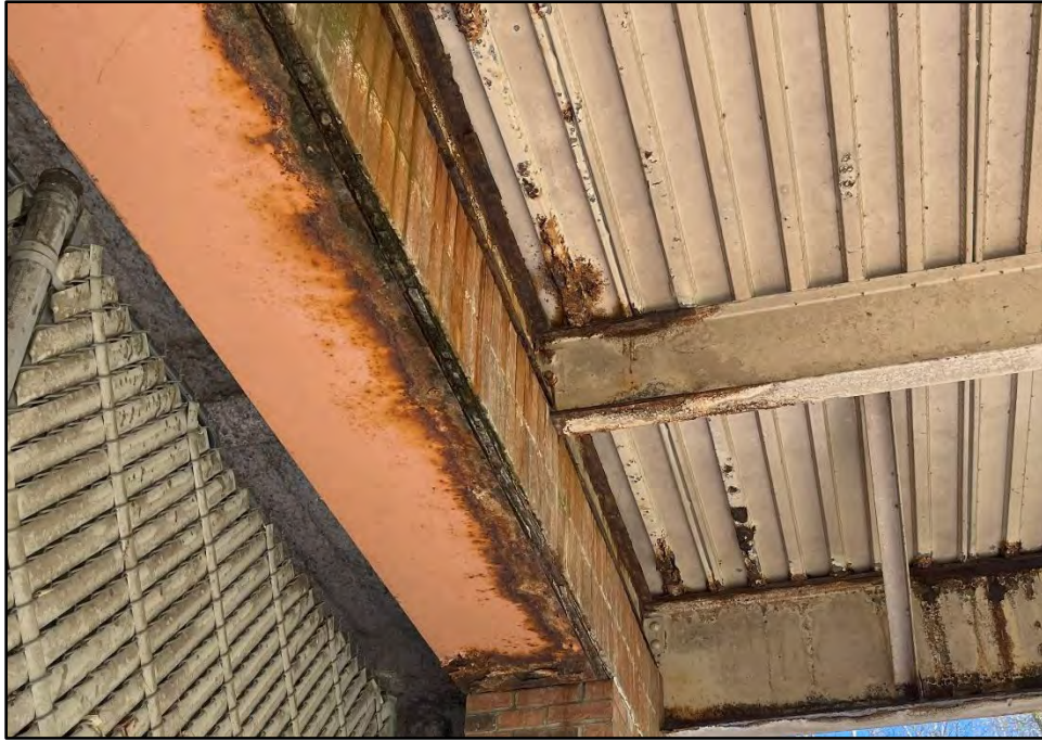
Image 16: Lintel Corrosion Under Raised Landing
