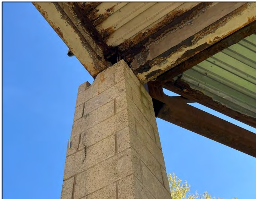
Image 15: Chipping of Masonry from Flooding
