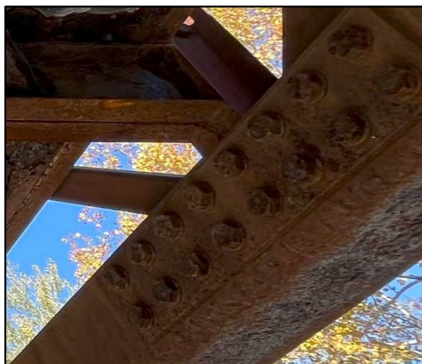
Image 12: Bottom Chord Splice Corrosion
