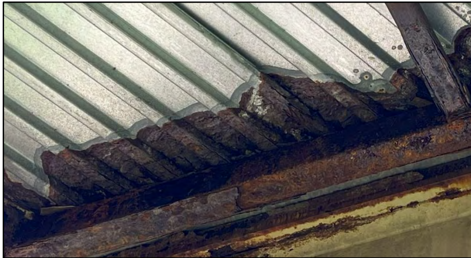
Image 10: Weathering Steel/Galvanized Deck Interaction
