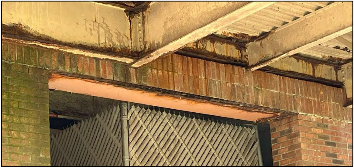
Image 14: North Landing Underside Corrosion
