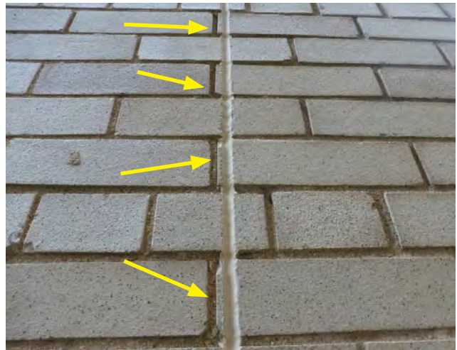
Photo 2 Poorly Aligned Remedial Expansion Joint
