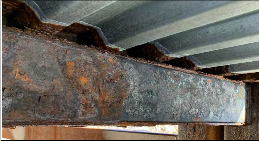
Image 2: Delamination Removed from Cross Member
