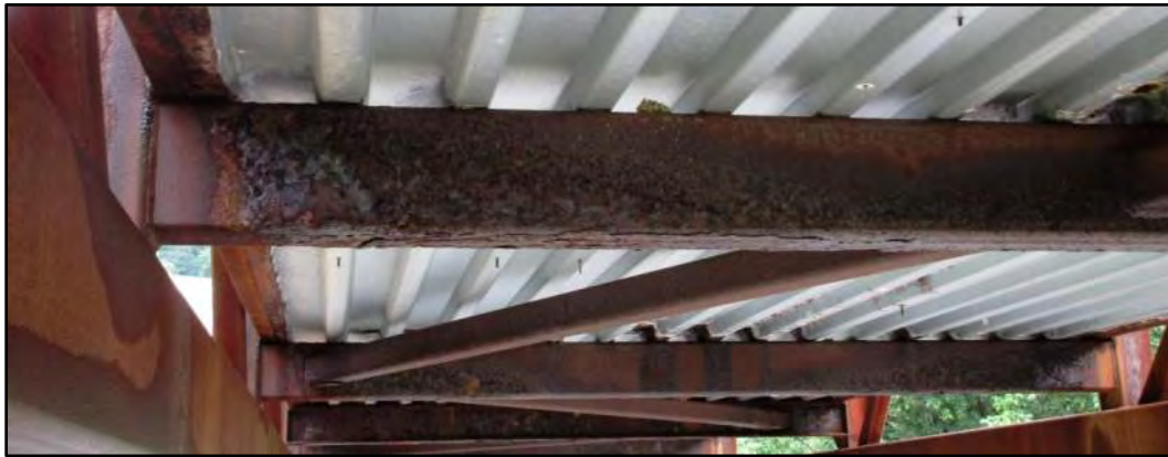
Image 9: Cross Member Corrosion
