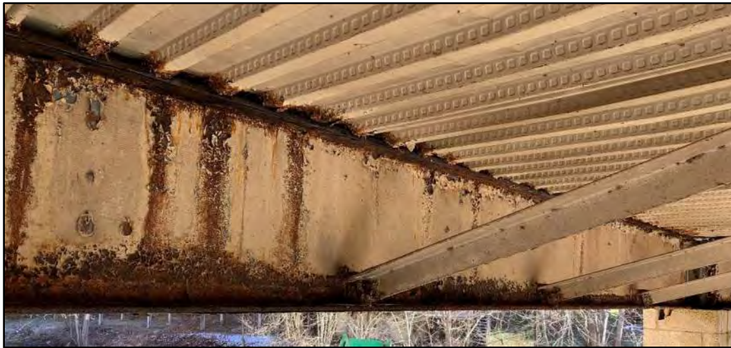
Image 16: North Landing Underside Corrosion
