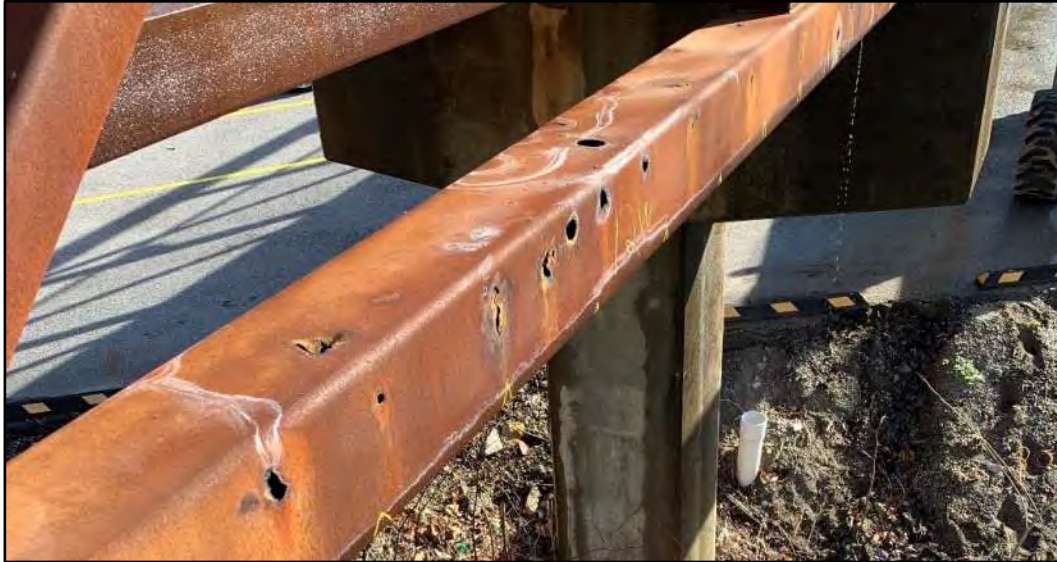
Image 6: Span 1, West Bottom Chord Deterioration
