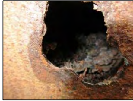
Image 7: Close-up of Holes through Bottom Chord
