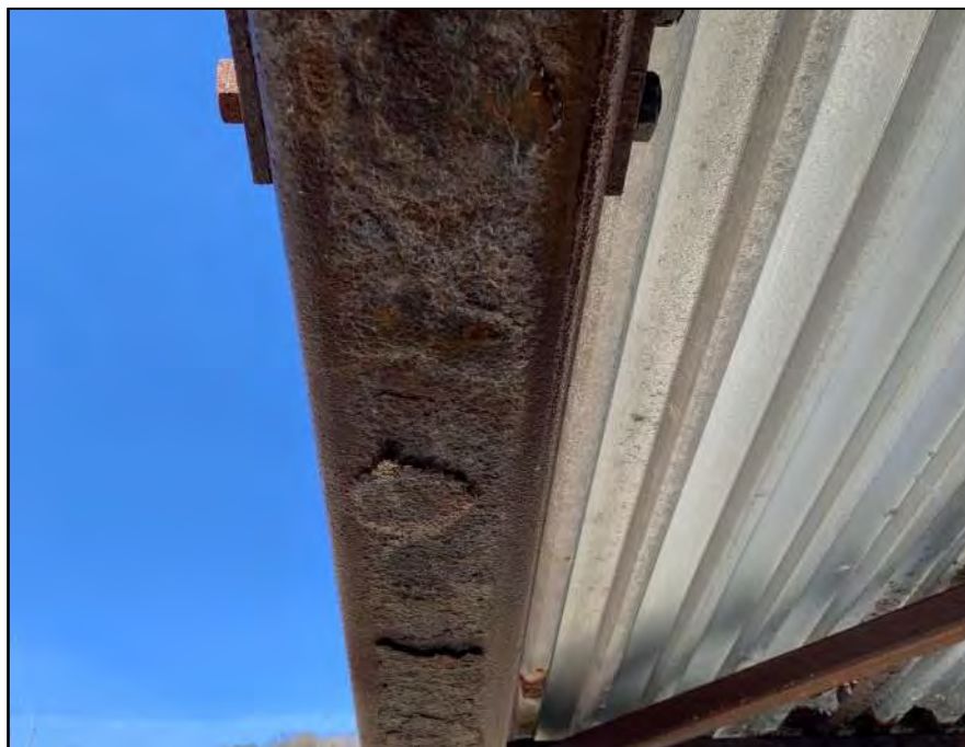
Image 8: Underside of Bottom Chord Delamination
