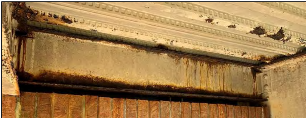
Image 17: Beam Corrosion at Building Intersection
