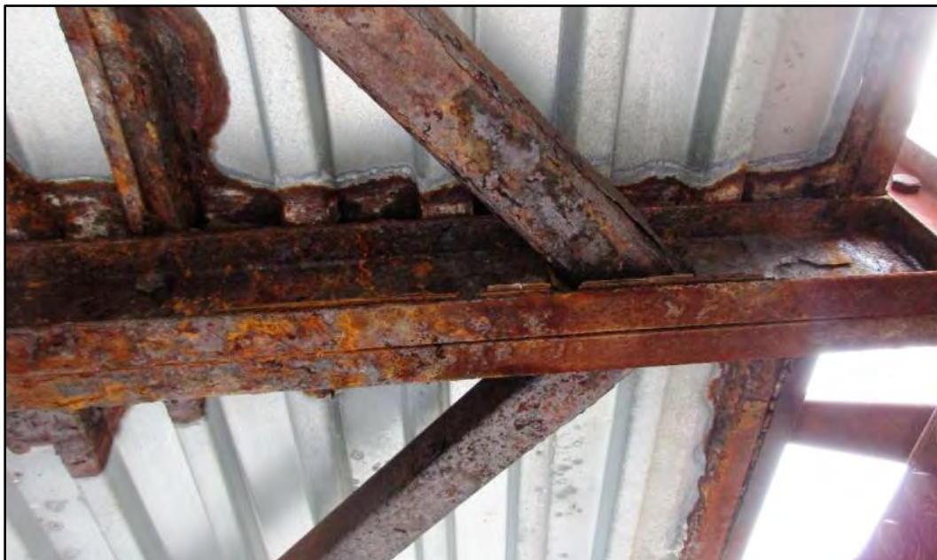
Image 10: Lateral Bracing Corrosion
