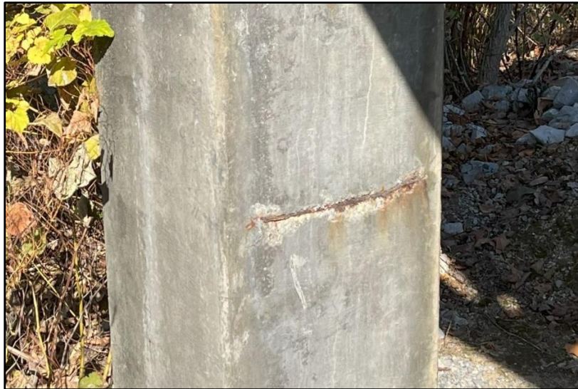
Image 11: Concrete Pier Spall
