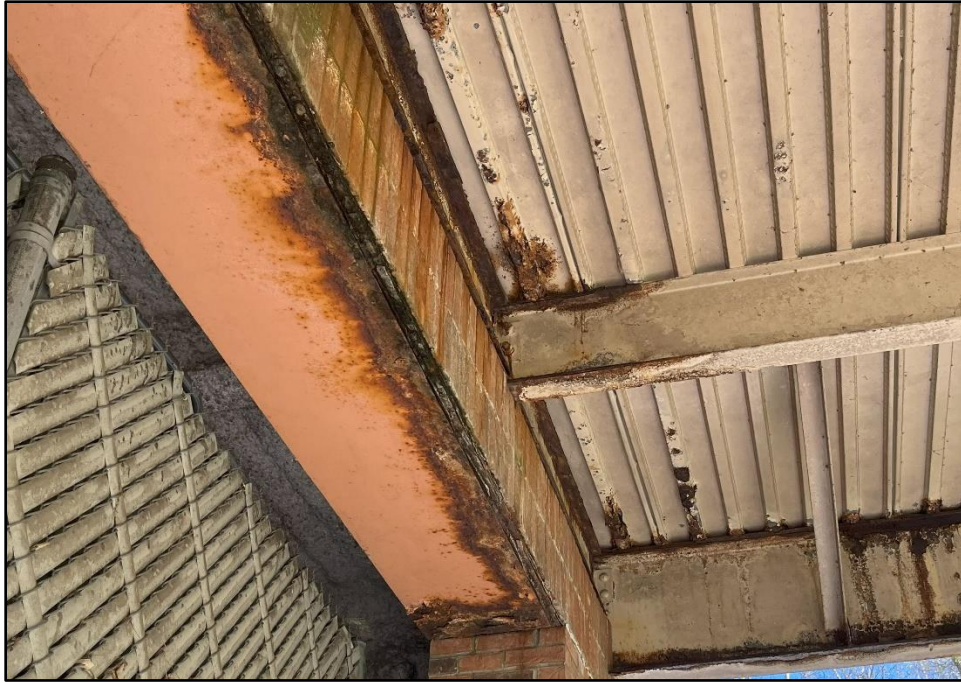
Image 16: Lintel Corrosion Under Raised Landing
