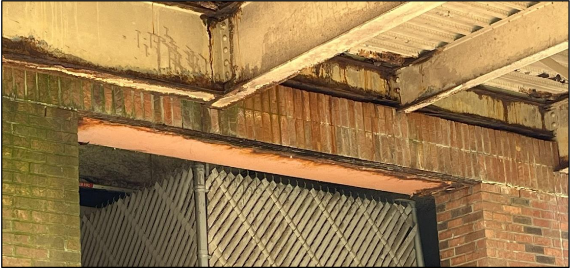
Image 14: North Landing Underside Corrosion
