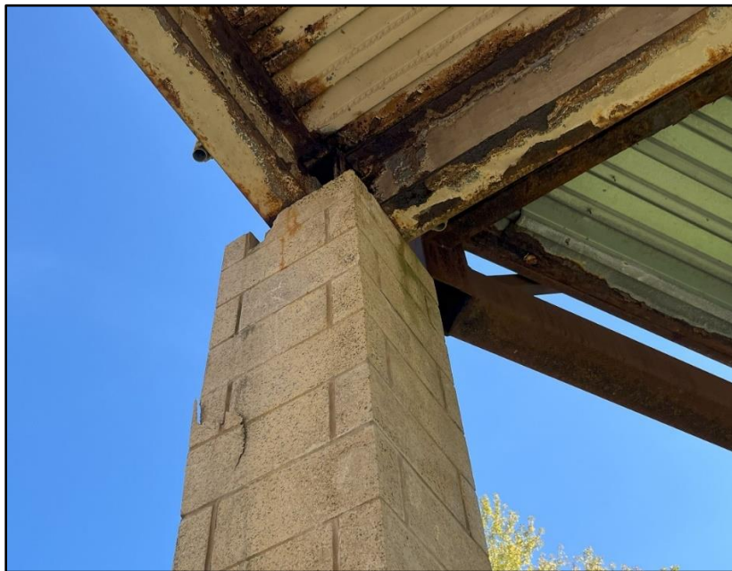
Image 15: Chipping of Masonry from Flooding
