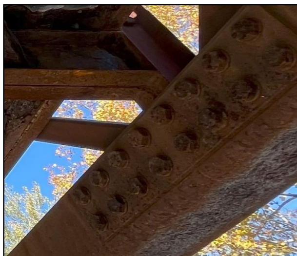
Image 12: Bottom Chord Splice Corrosion
