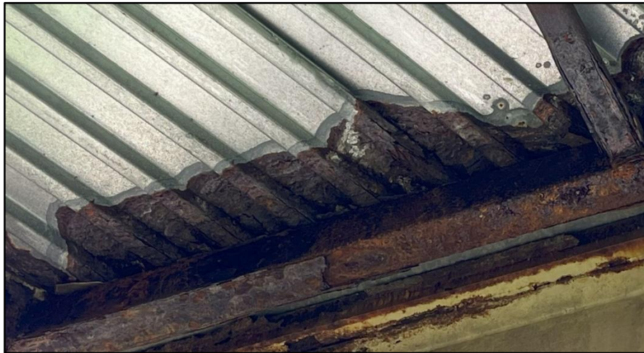
Image 10: Weathering Steel/Galvanized Deck Interaction
