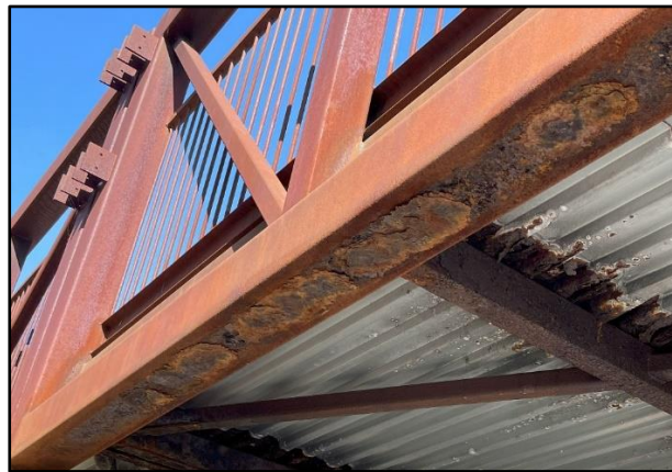
Image 7: Underside of Bottom Chord Delamination
